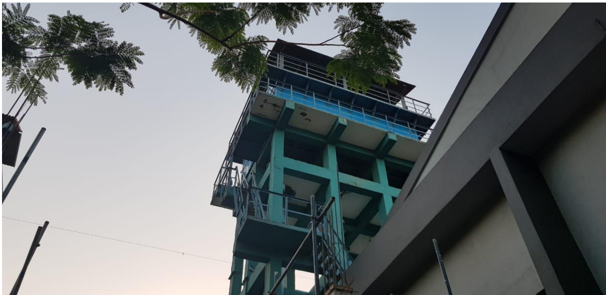
Fig 3.8 Over Head Water Tank used in the study with 17 m head
